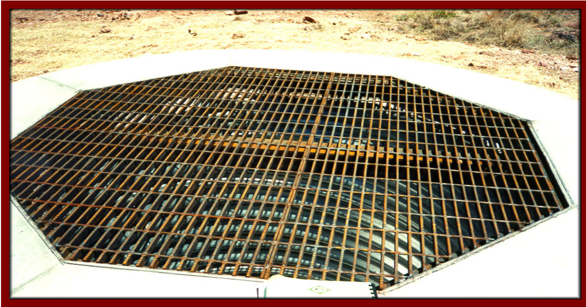
Close-up of the grated closure at the Feature 11 Shaft, showing the corrugated steel pipe riser (inside a polyurethane foam plug and masonry collar)
