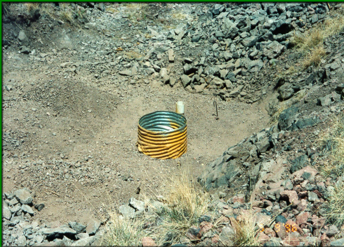
Corrugated steel pipe riser and polyurethane foam plug in place at the Feature 15 Shaft
