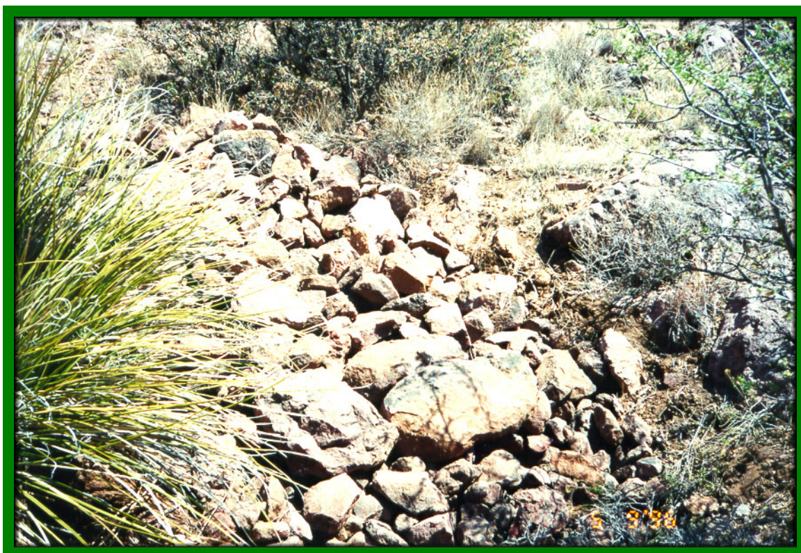
Feature 19 Adit backfilled with rock
