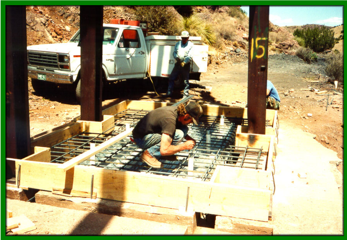
Constructed form for reinforced concrete slab at the Feature 4 Shaft
