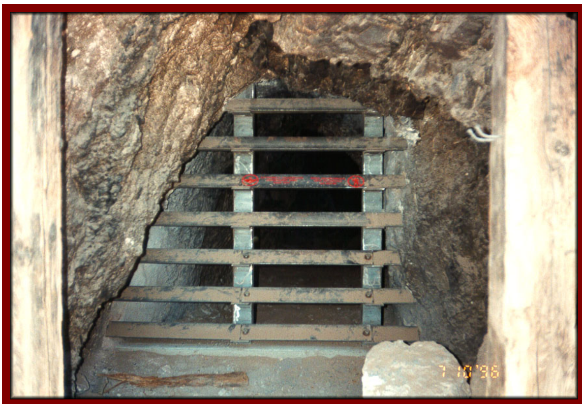
Completed bat closure in the Feature 7 Adit
