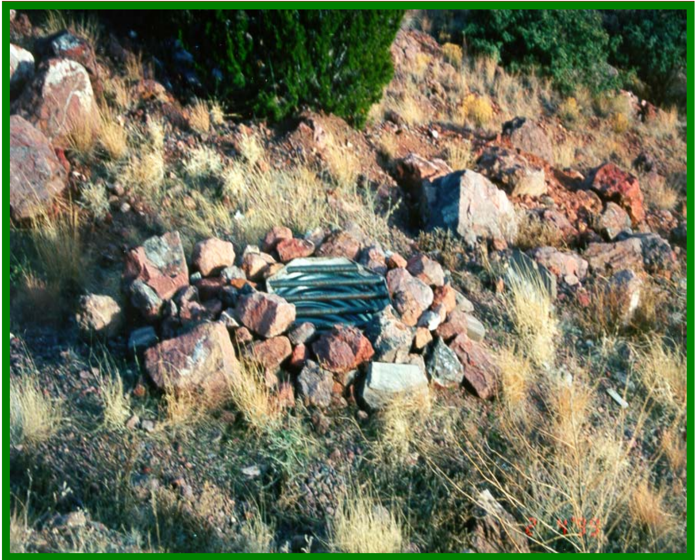
Feature 18 bat closure following vandalism, mortarless concrete units replaced with native rock
