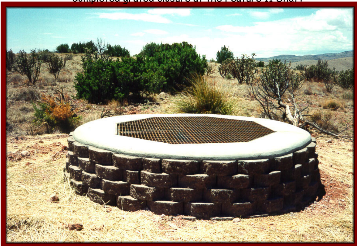
Completed grated closure at the Feature 11 Shaft
