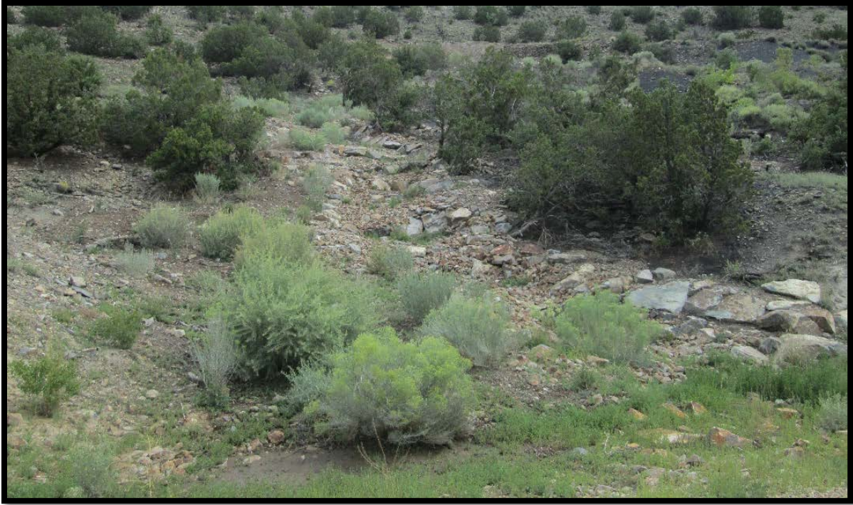
Figure 15. The completed step-pool rock bypass channel in August 2016. Note planted and seeded vegetation in and around the channel. The large light colored rock was covered with smaller tan rock to better blend channels into the surroundings.
