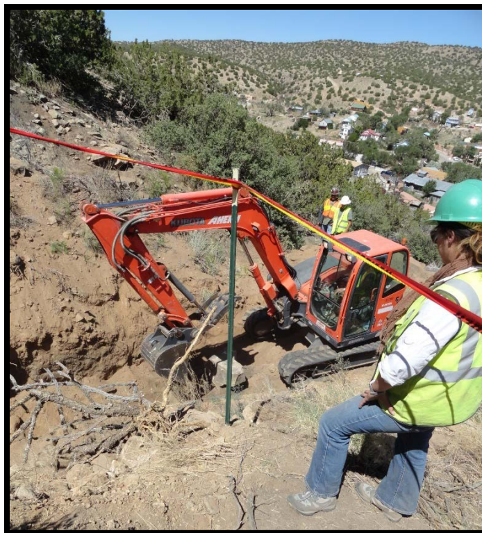
Figure 11. Backfilling the Cranky Charlie Coal Mine adit, June 2014
