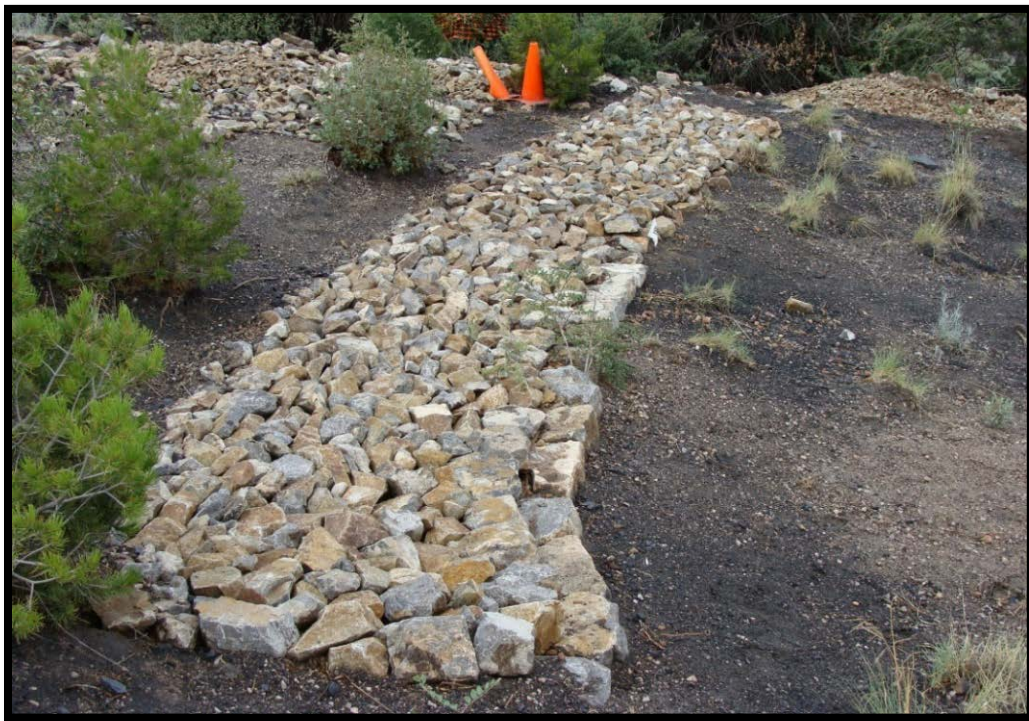
Figure 16. Newly constructed rock media luna on the larger gob pile to collect sheet flow, slow and infiltrate it, and direct it toward a rock mulch rundown below.
