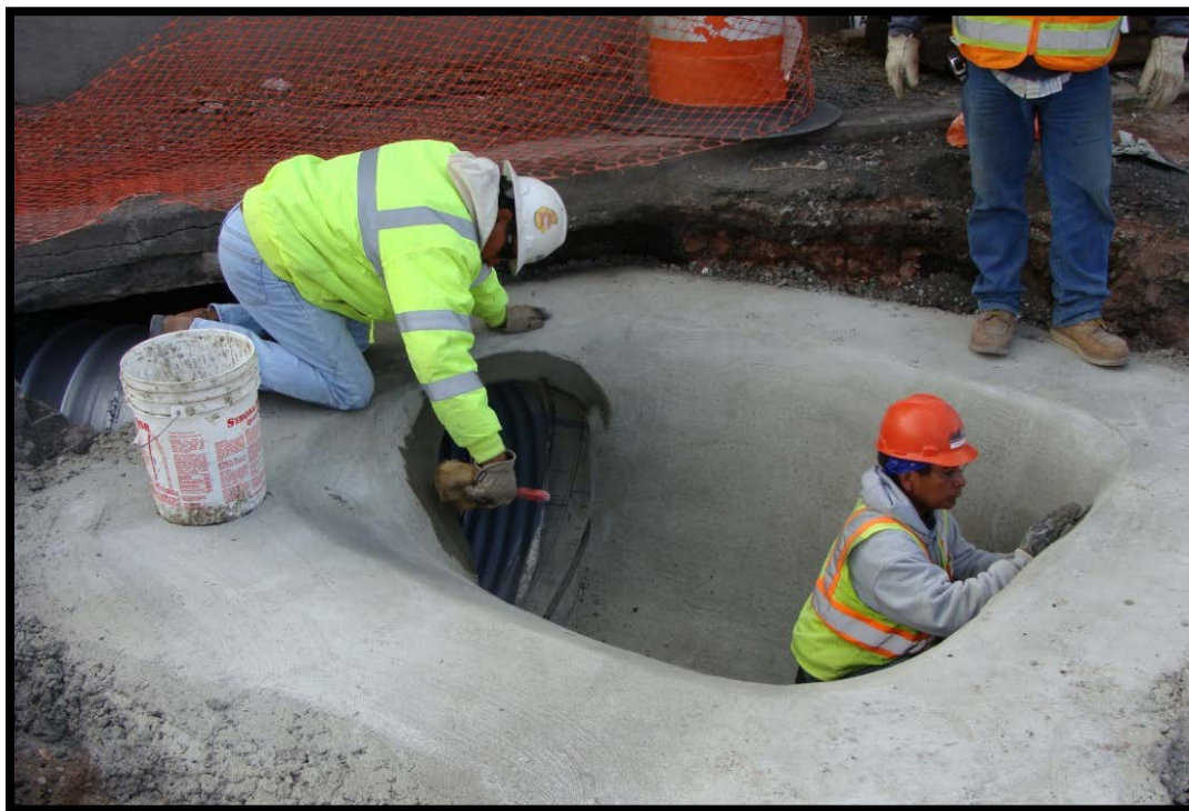
Figure 26. Casting new clean-out manhole immediately outside of the Mine Shaft Tavern (later capped with concrete slab with manhole ring and cover), March 2015
