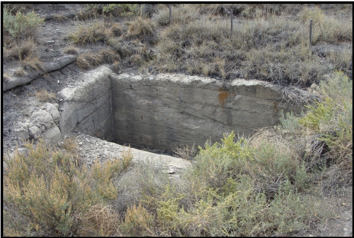
Figure 22. The derelict upper drop inlet below the gob piles and above the Museum before construction
