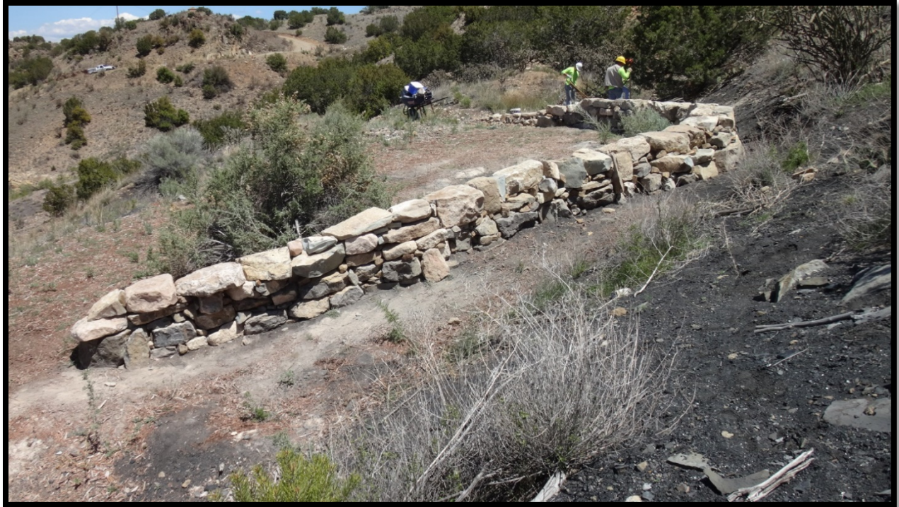
Figure 21. Raising of the dry stack rock wall to divert hillslope stormflows around the top of the larger reclaimed gob pile, May 2016
