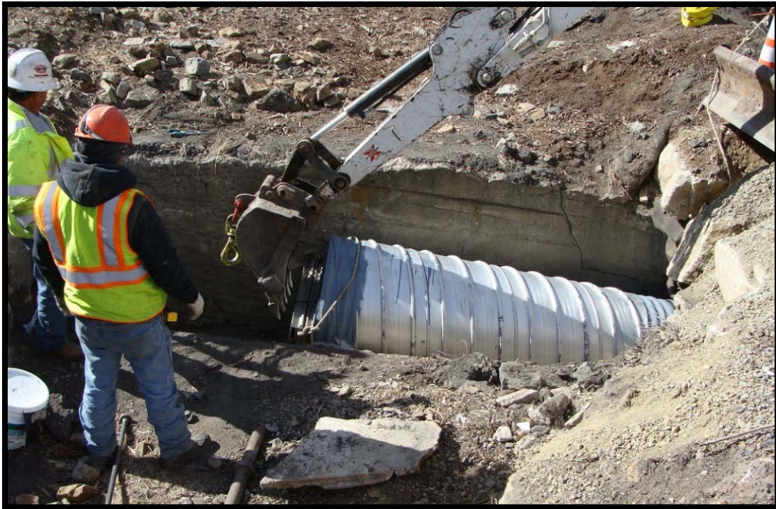
Figure 25. Sliplining 36-inch diameter steel pipe into the box culvert at the upper drop inlet, February 2015
