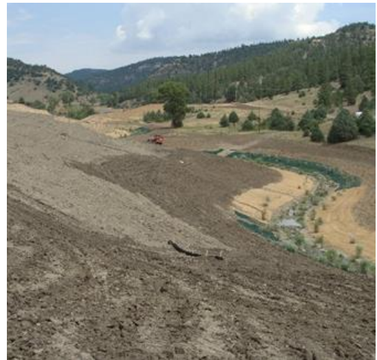
Newly planted vegetation and erosion protective fabric planted on the sides of the channel.
