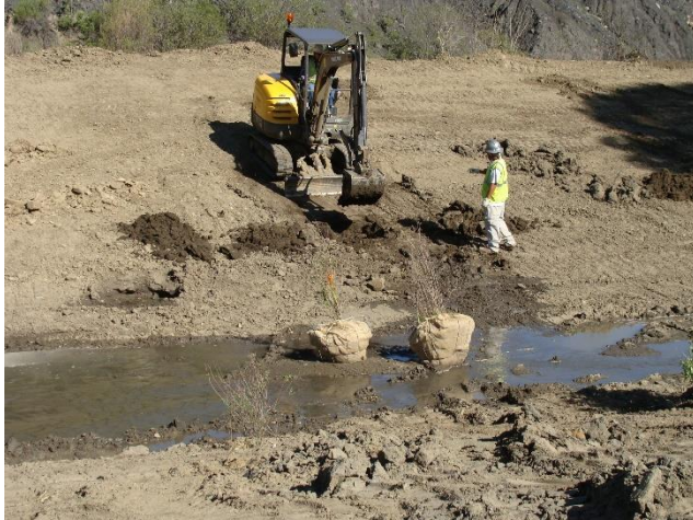
Planting willows and cottowoods in the newly constructed stream channel.
